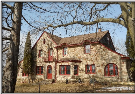
John and Razy Wright House, 1924 - This romantic style pseudo-Tudor home is located at W5670 CTH F in the Town of Medary. Its unique Flemish Bond stone exterior and arched windows and doorways were designed for the Wrights by regional artist Otto A. Merman.
